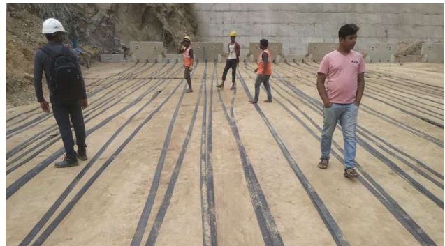
HIGHWAYS / ROAD CONSTRUCTION
